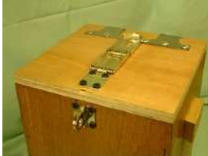
Figure 7 – Example box showing hasp and staple securing
